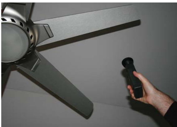
ST-1000 Checking Fan Speed and Balance
